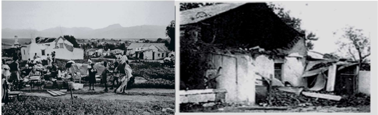
Figure 2.14 Damage observed at Tulbagh after the Ceres earthquake. Source: Pule et al. (2015). Adapted from Fernandez (1974).
