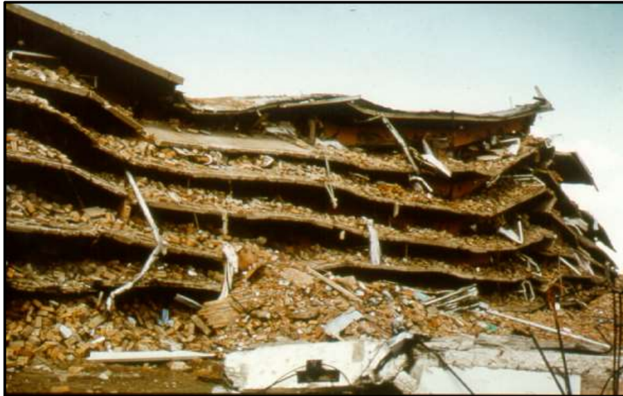
Figure 2.16 The collapse of six storeys apartment block was caused by the 1976 mining-related seismic event (Source: Council for Geoscience, Pretoria, photographer unknown).
