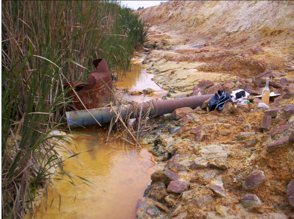
FIGURE 4: UNDESIGNATED UNDERDRAIN AT THE OLD TSF
