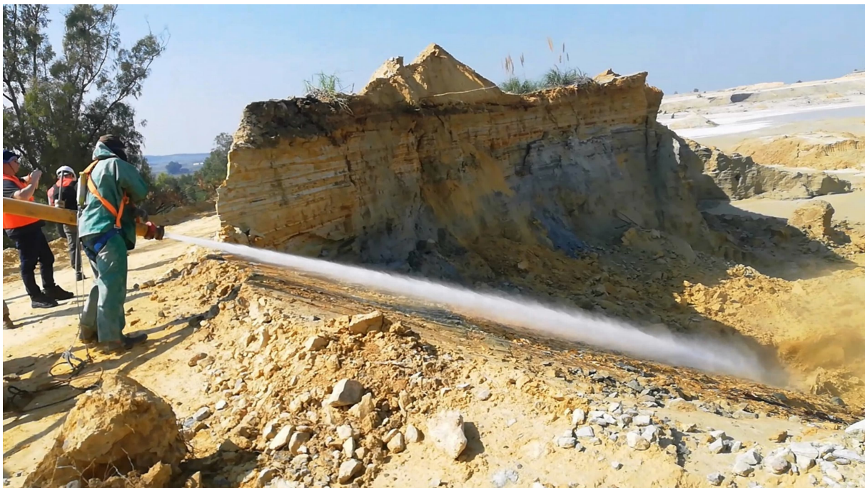
Figure 3-1: TSF 2 northern corner reclamation via high-pressure water jetting (26 March 2025)
