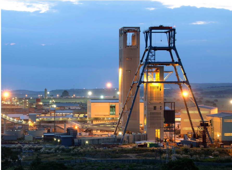
Figure 2.7 View of the Twin Shaft Complex of the South Deep Gold Mine, with the South Shaft Complex in the distance.
