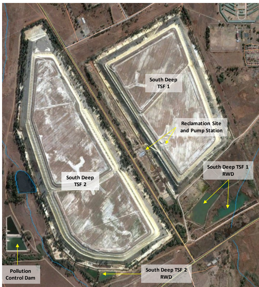
Figure 2.12 Google Earth view showing the two South Deep Gold Mine dormant TSFs, associated Return Water Dams, and the nearby-pollution control dam.
