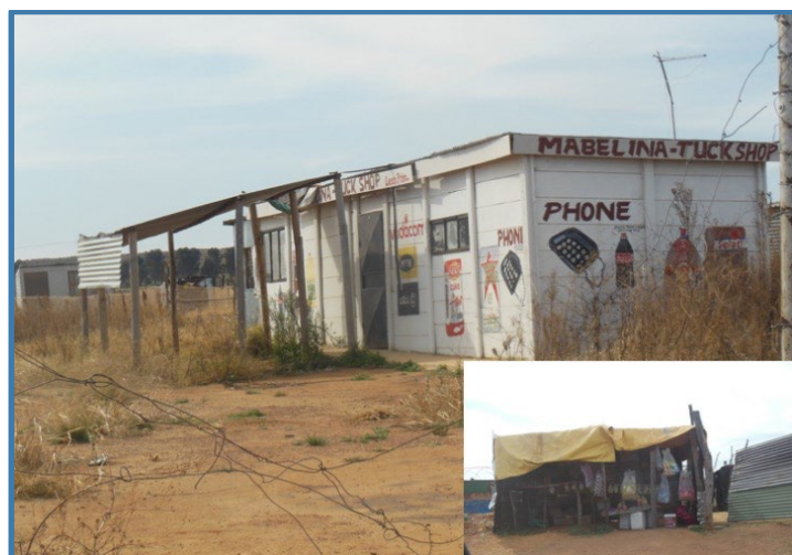
Figure 4.22 Shops in Thusanang (Equispectives, 2016).
