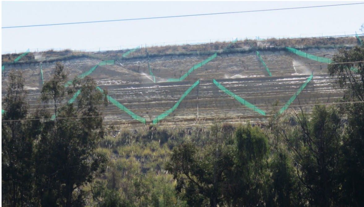
Figure 2.13 Netting, re-vegetation, and irrigation systems implemented at the two South Deep Gold Mine dormant TSFs.
