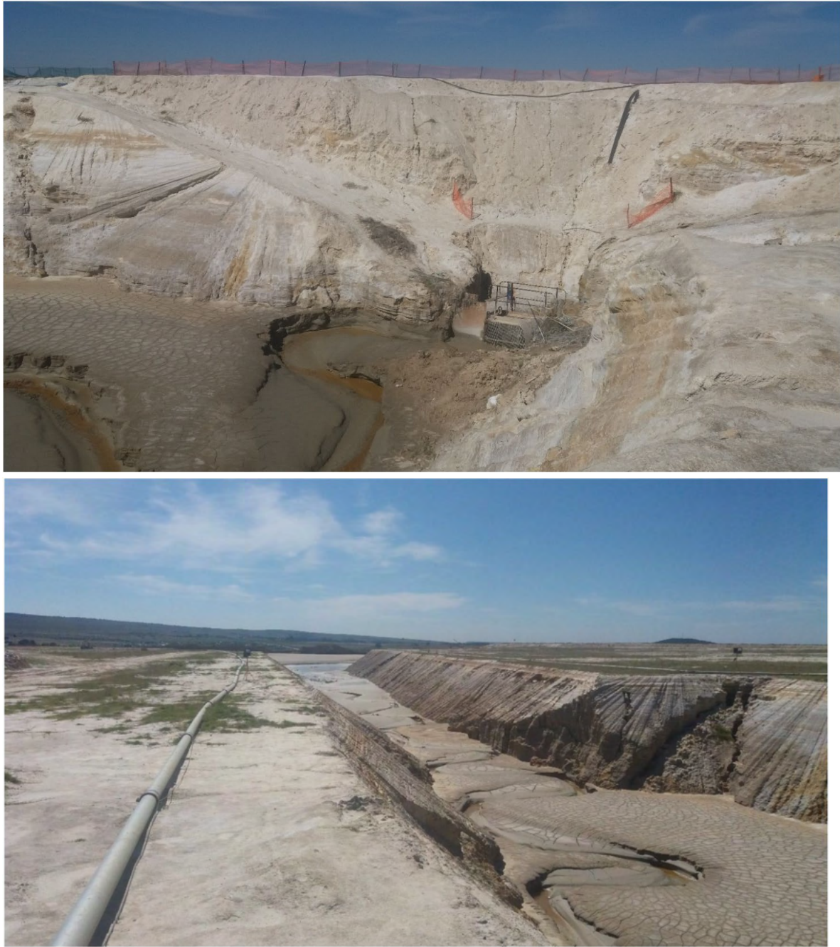
Figure 2.4 Photos showing the reclamation activities at the South Deep TSF 1 (Golder Associates, 2016).
