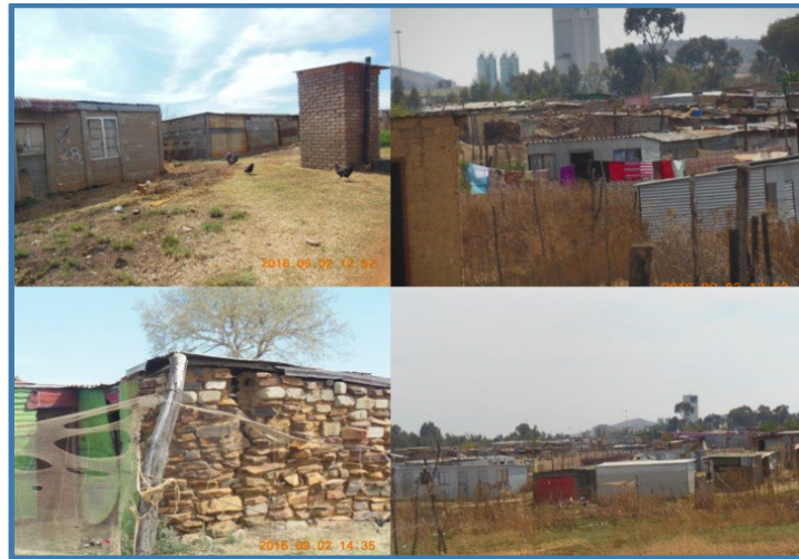
Figure 4.9 Dwellings in Thusanang, showing that most of the dwelling is constructed using Zinc (Equispectives, 2016).
