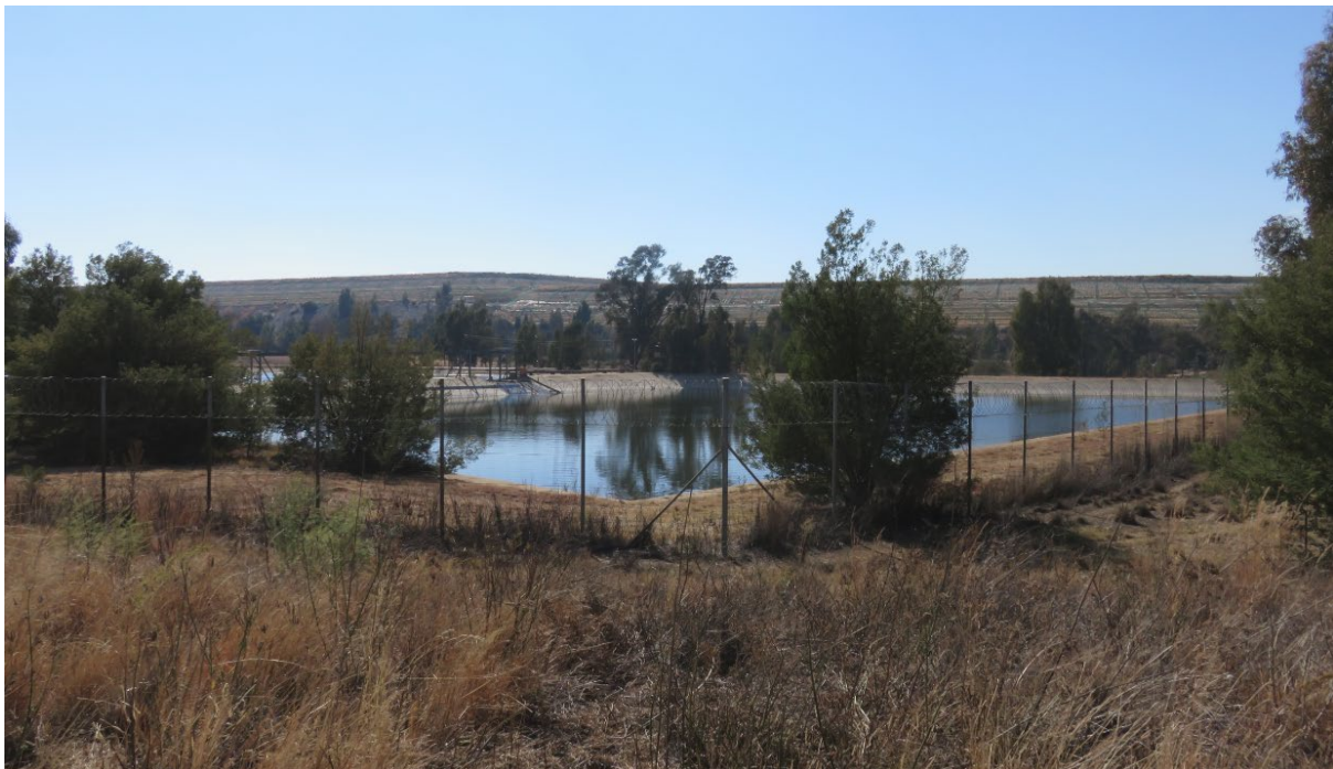
Figure 2.15 View of the concrete-lined Twin Shaft Complex pollution control dam.
