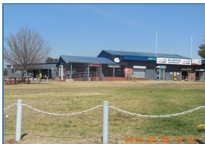
Figure 4.16 Supermarket in Hillshaven (Equispectives, 2016).
