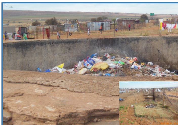
Figure 4.27 Refuse in old cement dam in Thusanang (Equispectives, 2016).
