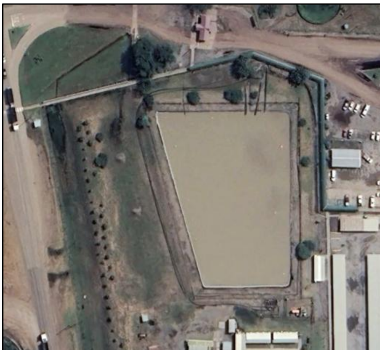
Figure 22: Process Water Dam
