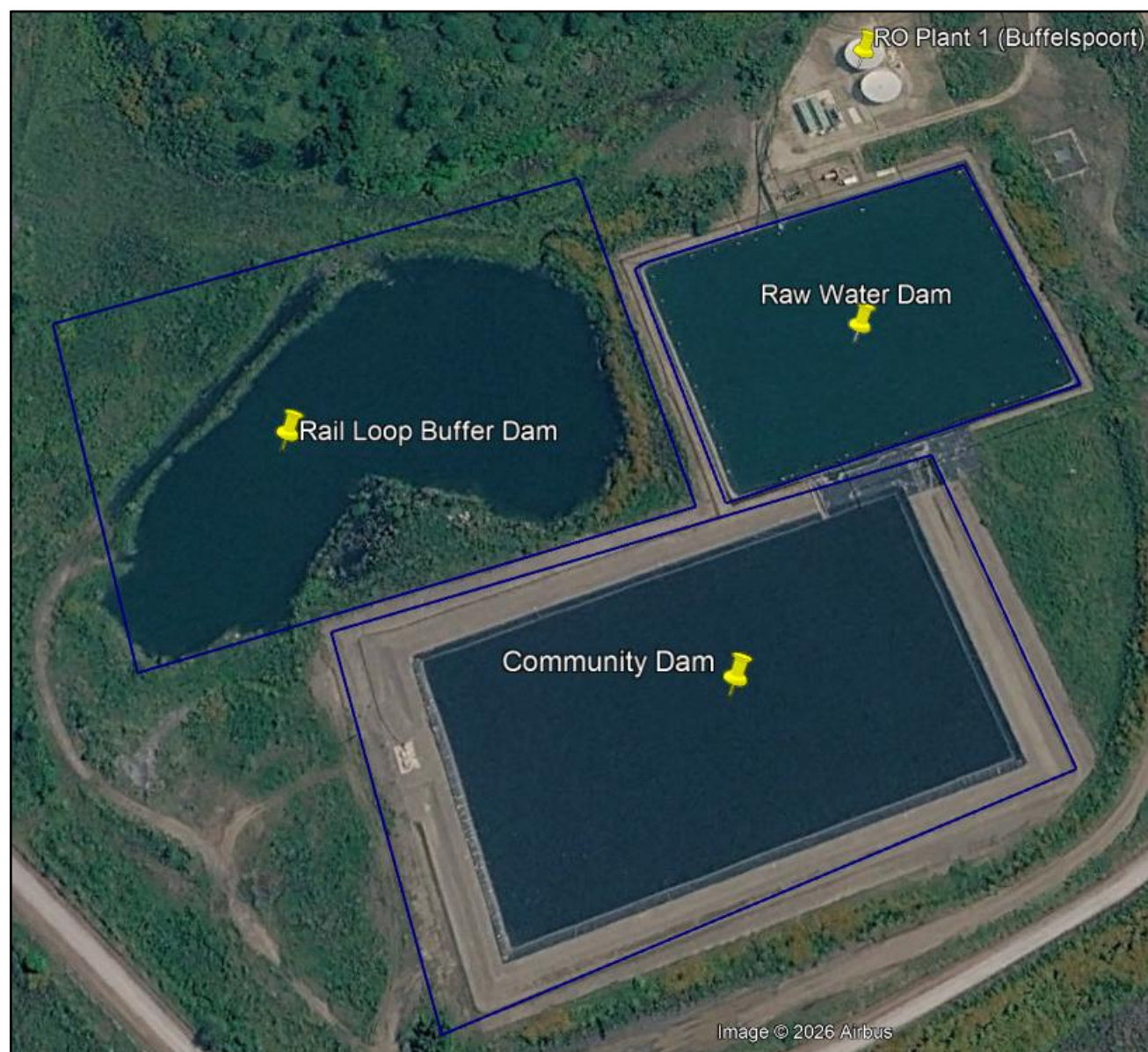
Figure 24: Raw Water Dam, Rail Loop Dam and Community Dam
