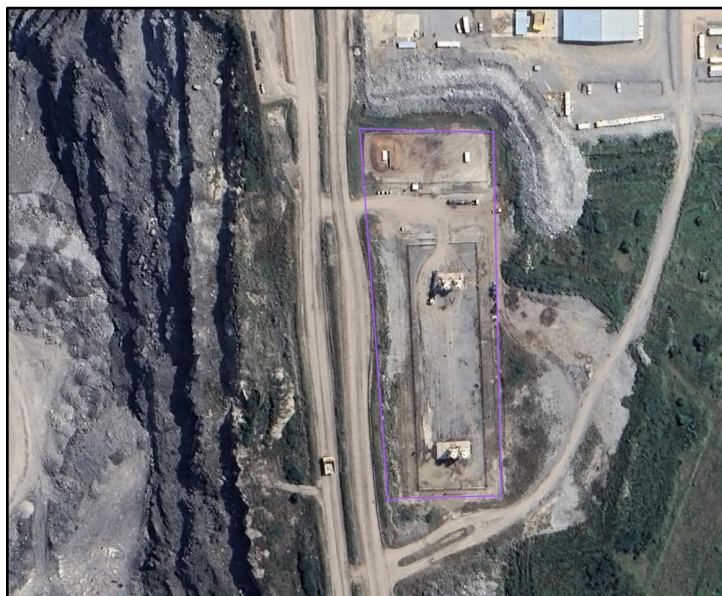
Figure 28: Explosive Magazine Storage and Emulsion Plant Area
